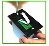
3.) Install the back side of your faceplate controller to the electrical box.
